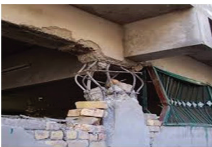
Fig.11: Failure due to Reinforcement deficiency at Gongabu
