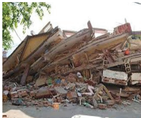
Fig. 6: Sandwich type failure at Sitapaila
