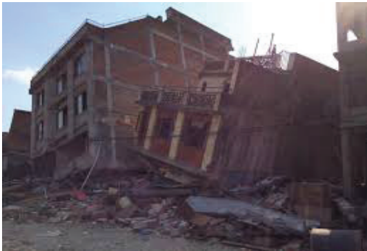
Fig.7: Soft storey failure at Gongabu
