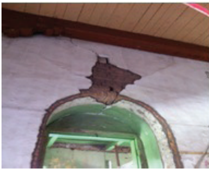
Fig.15: Damage on wall at the opening
