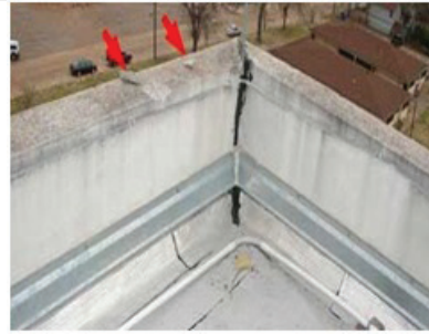
Fig.21: Damage on parapet wall at Katunje
