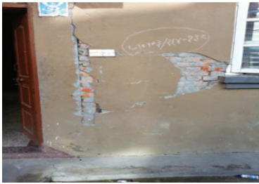
Fig.17: Damage at sill at Kirtipur
