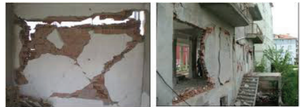
Fig.13: Damage on infill wall at Kavresthali
