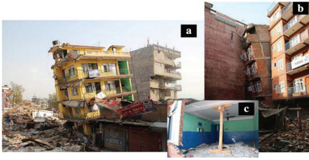
Fig. 3: At Gongabu, RC frame buildings were tilted (a, b). A shear crack in the first floor (c)
