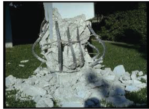
Fig.8: Crushing of concrete in column at Kalanki
