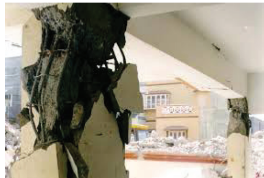
Fig.9: Shear and bending failure at Balaju
