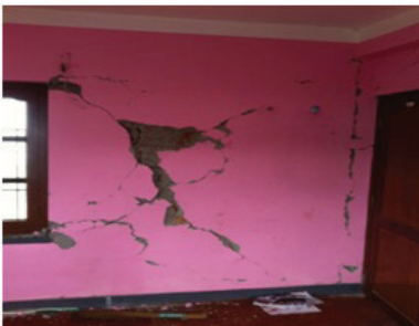
Fig.20: Damage on plaster at Balkot
