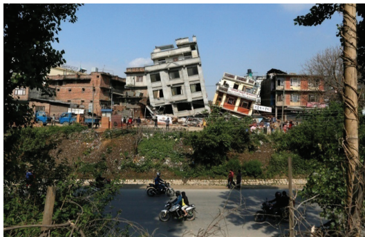
Fig. 4: Tilted building at Kalanki
