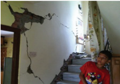
Fig.18: Damage at lintel at Goldhunga
