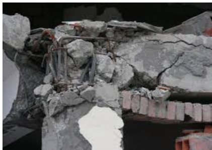
Fig.10: failure of beam column joint at Gongabu
