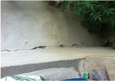
Fig.16: Damage on periphery at plinth at Mulpani
